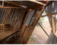
In February, a windstorm swept across the Rombo region of Kenya removing rooftops and causing the partial collapse of the Maasai Boma School wooden classroom structure. The Pillar of Maasai Development and school leadership are looking for financial help to repair the damaged building at an estimated cost of \$2000.
